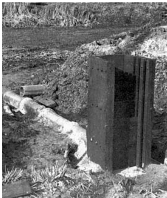
Fig. 6.8 Monks made of concrete (above) and wood (below). Outlet pipe can be seen behind the wooden monk. (From Huet, 1986.)
