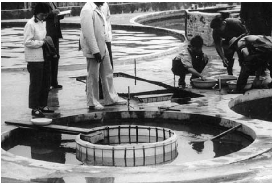
Fig. 6.20 Circular tanks in a Chinese fish-breeding station. Inlet nozzles (arrow marks on the walls show their positions) ensure proper water circulation.
