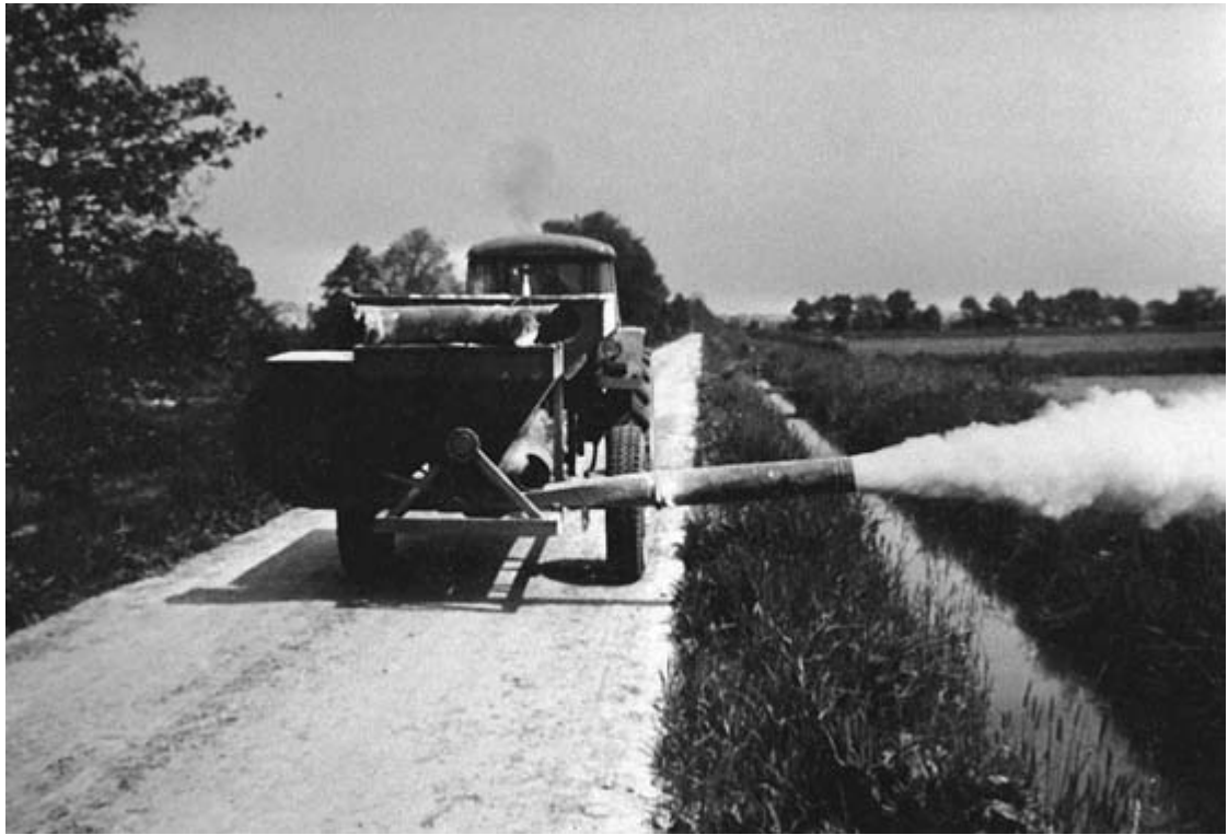
Fig. 7.15 A blower tank for dispensing feeds.
