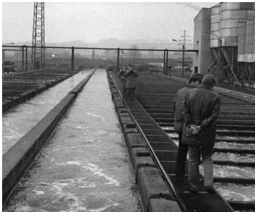
Fig. 6.21 A tank farm with cement-concrete rectangular tanks arranged on the side of the water supply system. Note the rails on the side of the tanks for transporting feed and the silos on the right for feed storage. (Courtesy of J. Kovari.)
