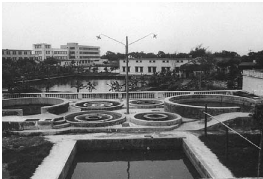
Fig. 16.20 Incubation and hatching pools: note the concentric multiple chambers in the pools in the centre.
