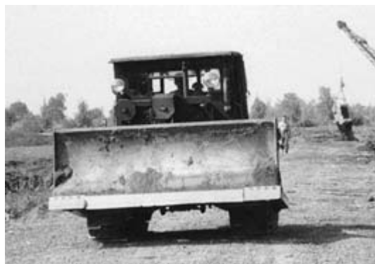
Fig. 6.13 Bulldozer used for pond construction. (Courtesy of J. Kovari.)
