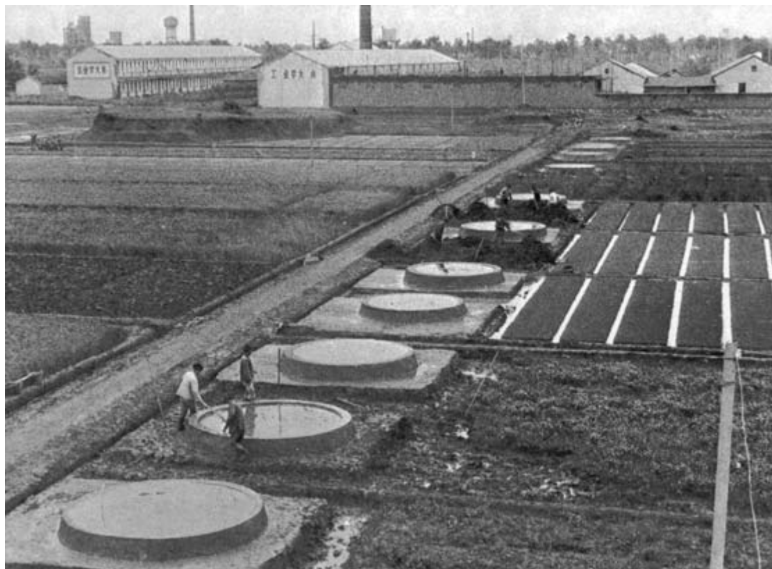
Fig. 7.4 Cement concrete pits used for composting silt, rice straw and animal manure in China. (From FAO Soils Bulletin, 40.)
