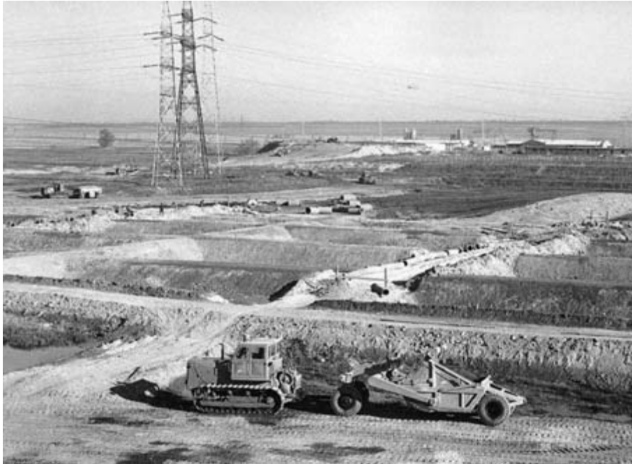
Fig. 6.14 Tractor-driven scrapers being used in pond construction. (Courtesy of J. Kovari.)
