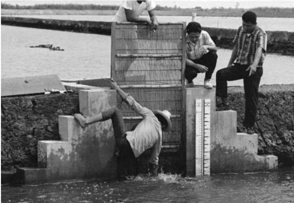
Fig. 6.9 Concrete sluice gate for a tidal pond farm in the Philippines. Note the bamboo screen.
