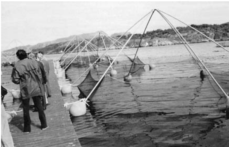
Fig. 6.27 A farm in Norway, which uses a different design of floating six-sided cages. Flotation is provided by six inflatable rubber buoys kept in place by six fiberglass poles radiating from a steel plate above the cage, looking like an inverted umbrella frame.
